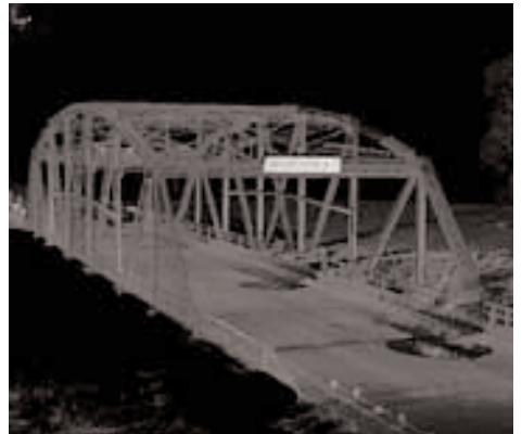
Twelve million data points capture this image of a truss bridge.
